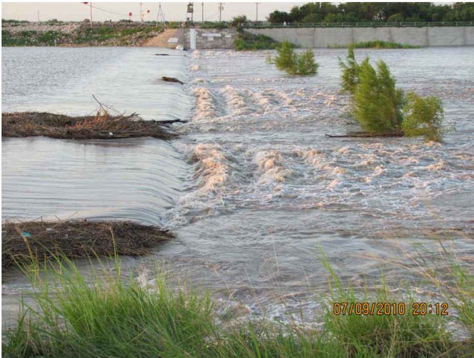
Gaging station at Banker Weir Inlet
