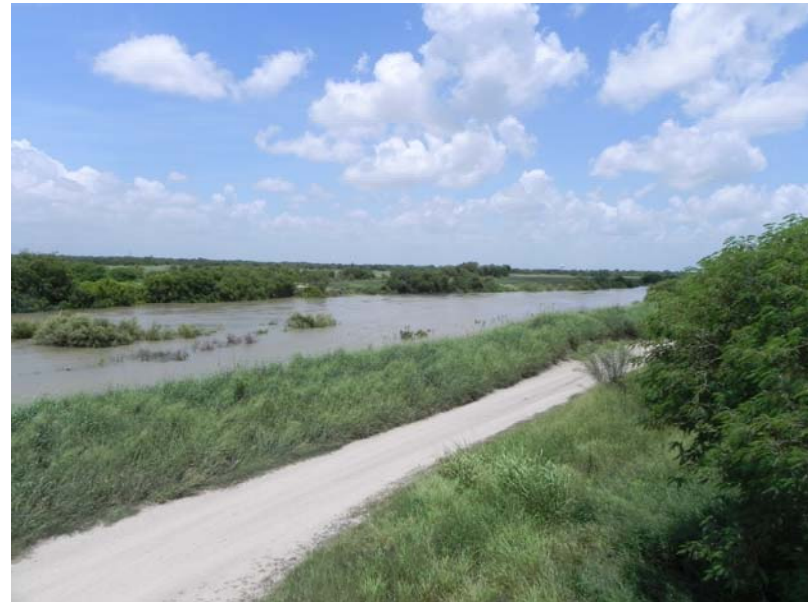
Rio Grande levee near Brownsville, 7/19/10
